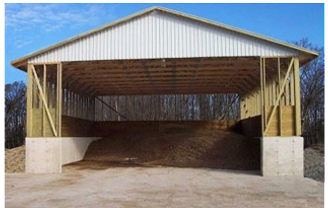
A covered manure storage eliminates runoff.
