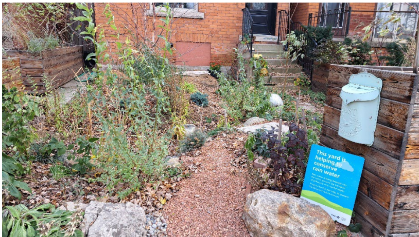
A completed rain garden in urban Hamilton.
