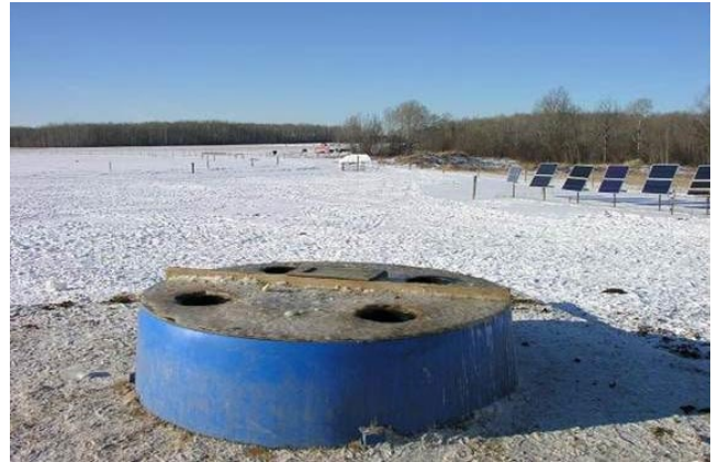
Insulated water trough with solar panels at right. © Queen's Printer for Ontario, 2016
