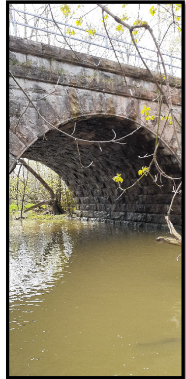
Photo 7: Trail Bridge over Welland River
