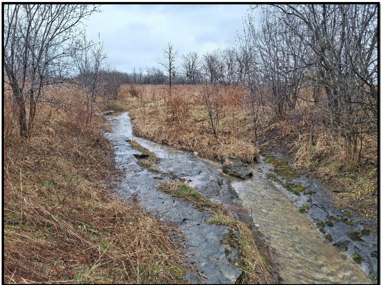
Photo 14: Water flowing into the Nexus Cave entrance after rainfall
