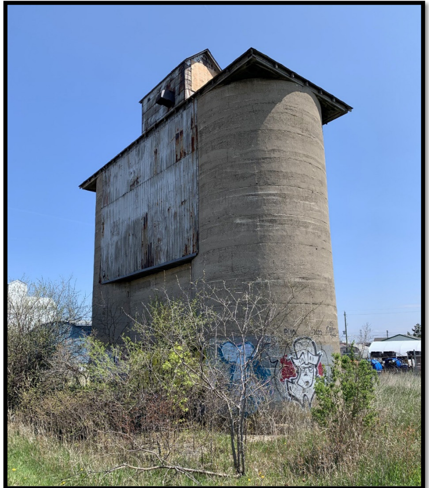
Photo 3: Former Harris Grain Elevator
