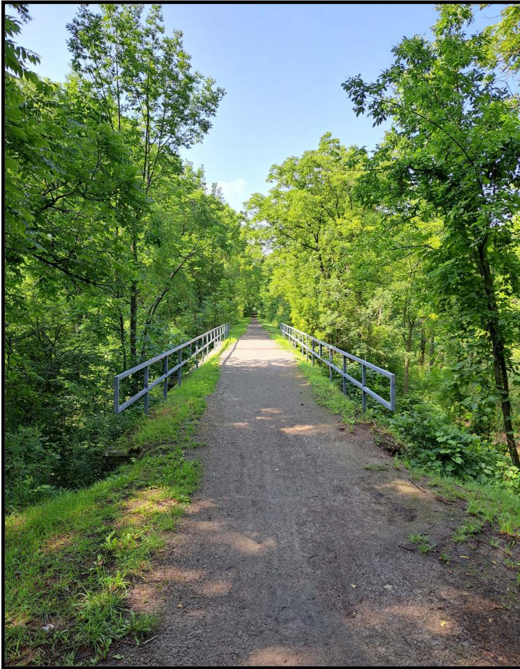
Photo 17: Chippawa Trail bridge over Twenty Mile Creek
