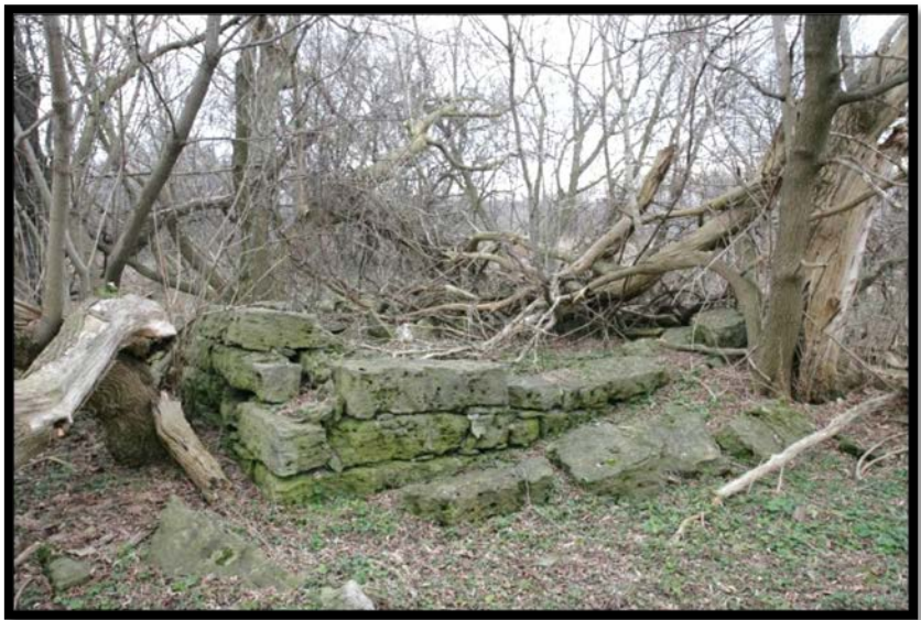
Photo 20: Remaining foundations at the Pottruff site.
