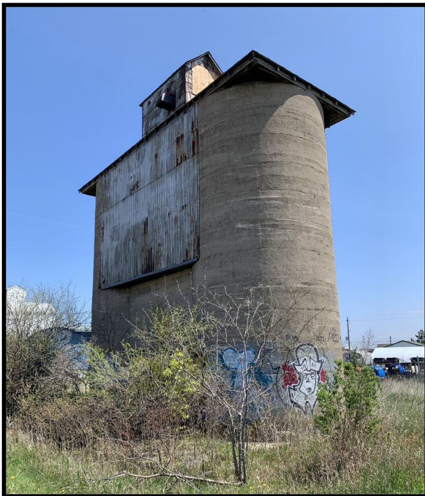
Photo 3: Former Harris Grain Elevator
