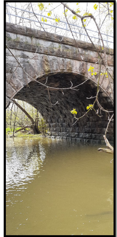
Photo 7: Trail Bridge over Welland River
