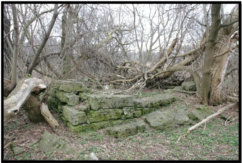
Photo 20: Remaining foundations at the Pottruff site.
