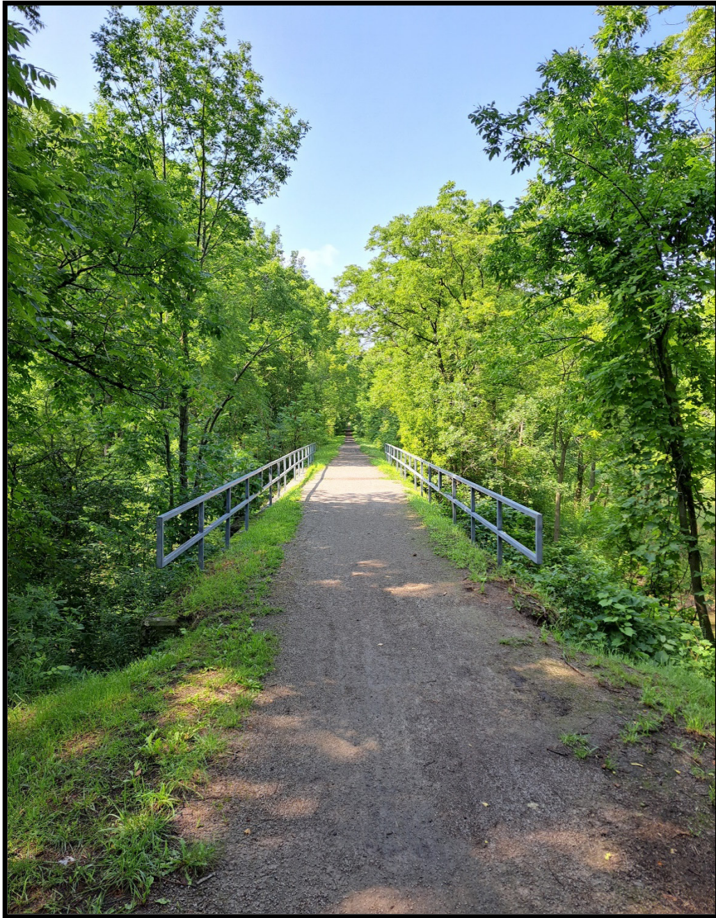
Photo 17: Chippawa Trail bridge over Twenty Mile Creek
