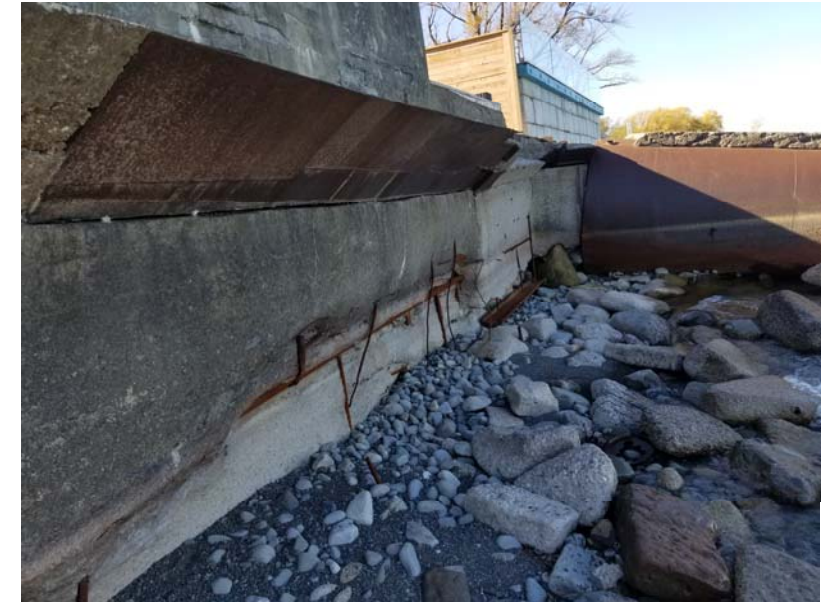
Evidence of Exposed Reinforcements and Scour at Toe
