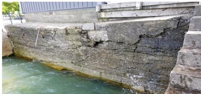
Figure 4: Existing fractured Seawall of the Property (Facing North)
