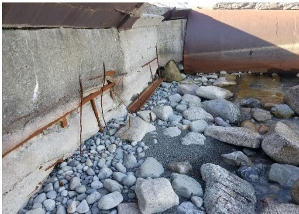
Figure 9: Exposed Reinforcement of the Concrete Seawall at the Shoreline with Washed out Small and Medium Stones at the Toe
