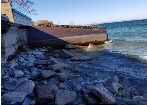
Figure 7: Existing Steel Barrel Groyne
