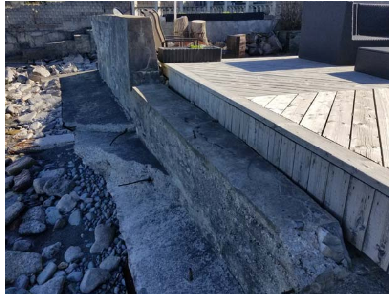
Condition of Existing Concrete Seawall in front of 10 Lakeside Drive Property
