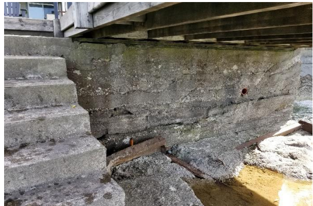
Figure 4: Exposed steel sheet piles
