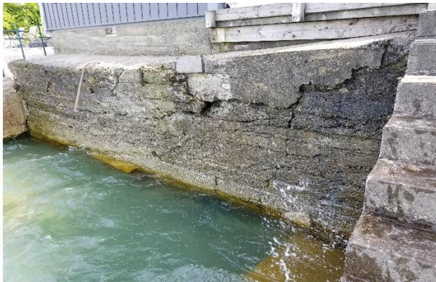
Figure 3: Fractured Seawall at right side of deck
