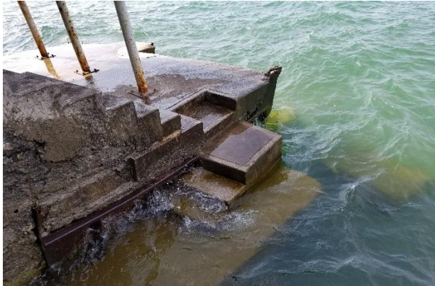
Figure 7: Fallen Concrete blocks underwater
