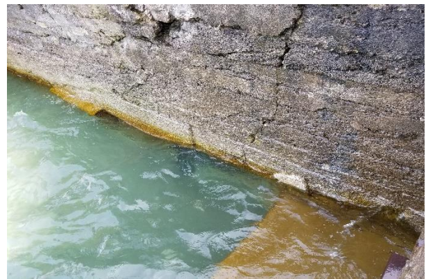
Figure 6: Scour under existing seawall
