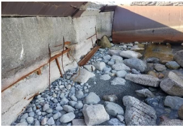
Figure 5: Condition of the toe of the existing seawall
