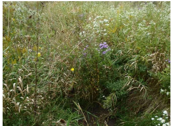
Photo 35: Erosion along property boundary from feature being moved
