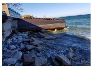
Figure 7: Existing Steel Barrel Groyne
