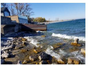
Figure 6: Shoreline in front of the Property with Existing Seawall and Steel Barrel Groyne
