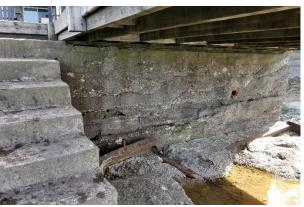
Figure 4: Exposed steal sheet piles
