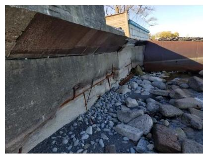
Evidence of Exposed Reinforcements and Scour at Toe
