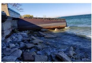
Figure 6: Existing steel barrel groyne at the western side of the property
