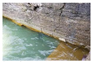
Figure 6: Scour under existing seawall
