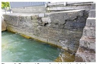
Figure 3: Fractured Seawall at right side of deck
