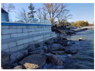
Figure 10: Seawall of Neighbouring Property at Left with Large Armourstones used as Toe Protection
