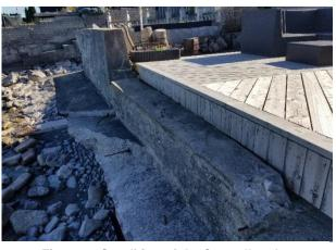
Figure 8: Condition of the Seawall at the Shoreline in front of the Wooden Deck
