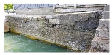
Figure 4: Existing fractured Seawall of the Property (Facing North)
