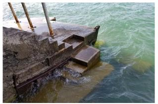
Figure 7: Fallen Concrete blocks underwater
