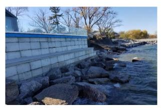
Figure 8: Shoreline of the neighbouring property at left with a newly built seawall and toe protection
