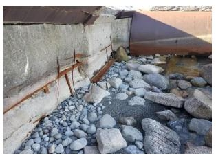
Figure 9: Exposed Reinforcement of the Concrete Seawall at the Shoreline with Washed out Small and Medium Stones at the Toe
