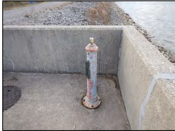
Photo 6 – Low Flow Valve Stem
