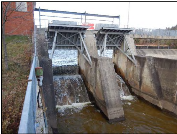
Photo 5 – Main Spillway Gates
