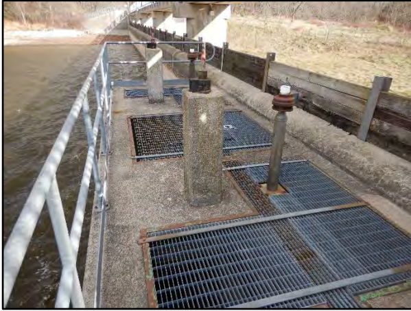
Photo 9 – Drop Inlet Structure Deck
