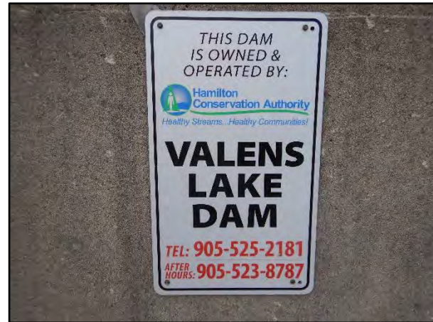
Photo 14 – Typical Inlet Structure Sign
