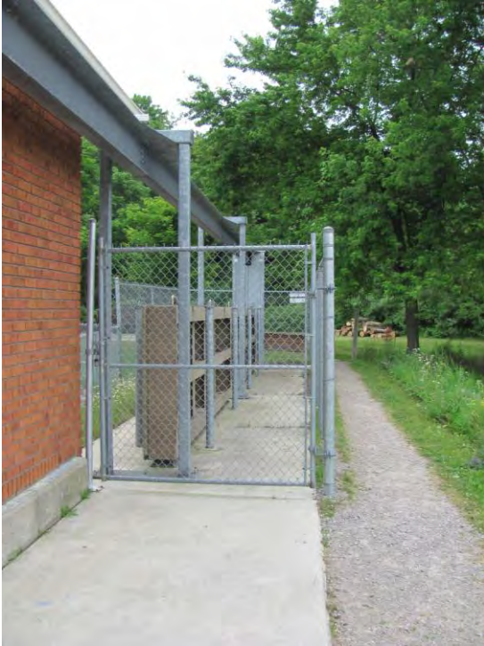
Photo 17: Steel panels storage area (July 2011)
