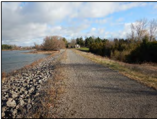
Photo 1 – Access Road Across Dam
