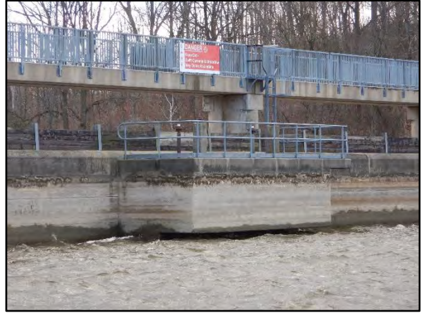
Photo 10 – Drop Inlet Structure
