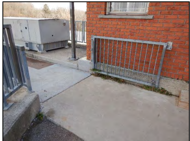
Photo 30 – Typical Pedestrian Barricade
