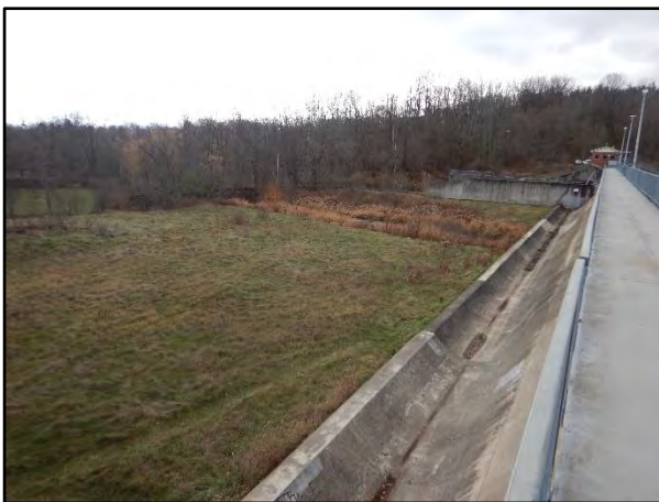
Photo 13 – Emergency Spillway
