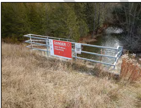
Photo 17 – Outlet Structure Railing
