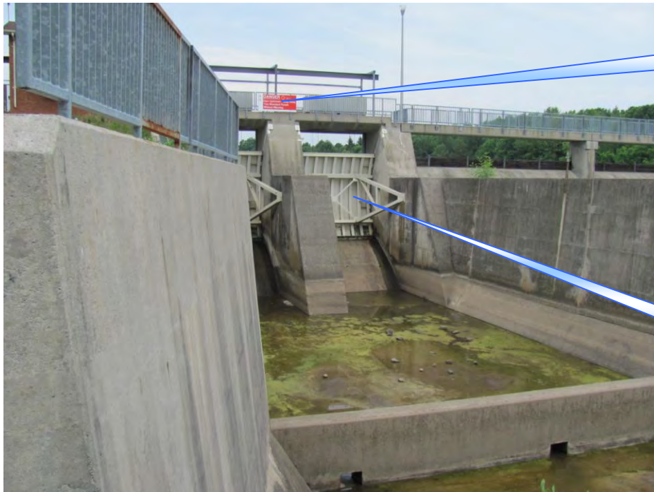
Photo 6: View of upstream face of ogee weir (April 2011)
