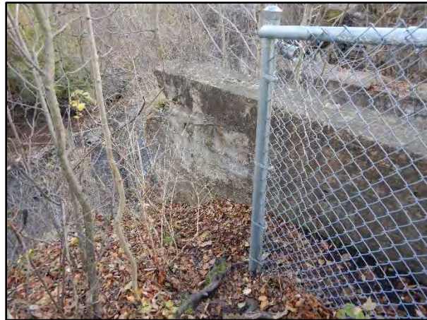
Photo 43 – End of Exterior Fencing
