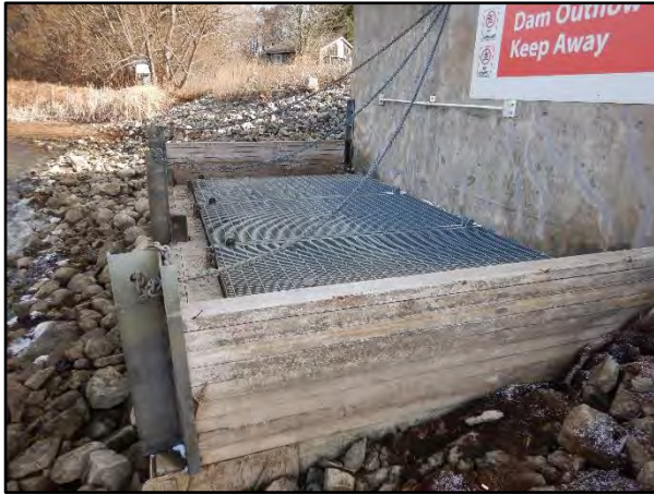
Photo 5 – Concrete Inlet Structure
