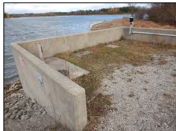
Photo 18 – Inlet Structure Barricade
