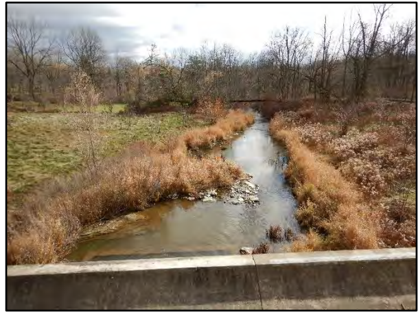
Photo 12 – Low Flow Channel
