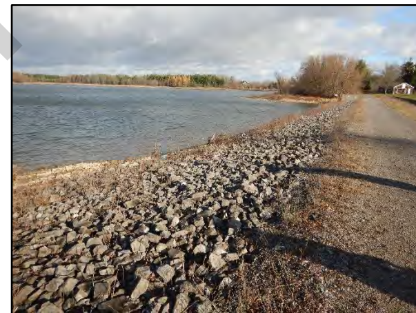
Photo 4 – Upstream Earth Embankment
