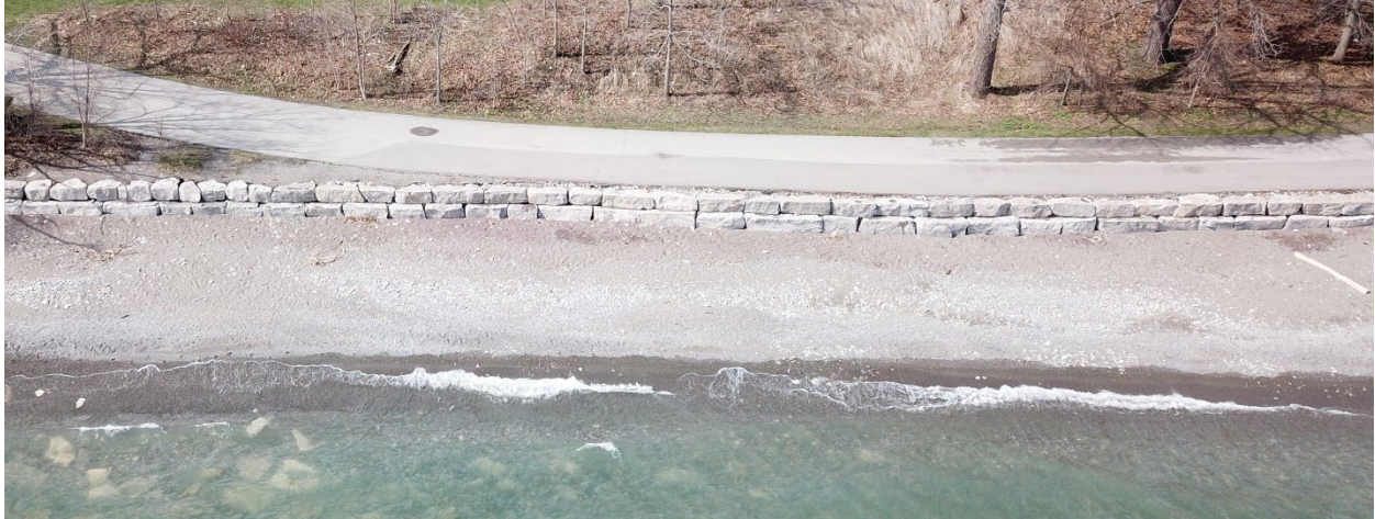
Figure 7.15 Example of a stacked armour stone beach curb at Confederation Park, Hamilton
