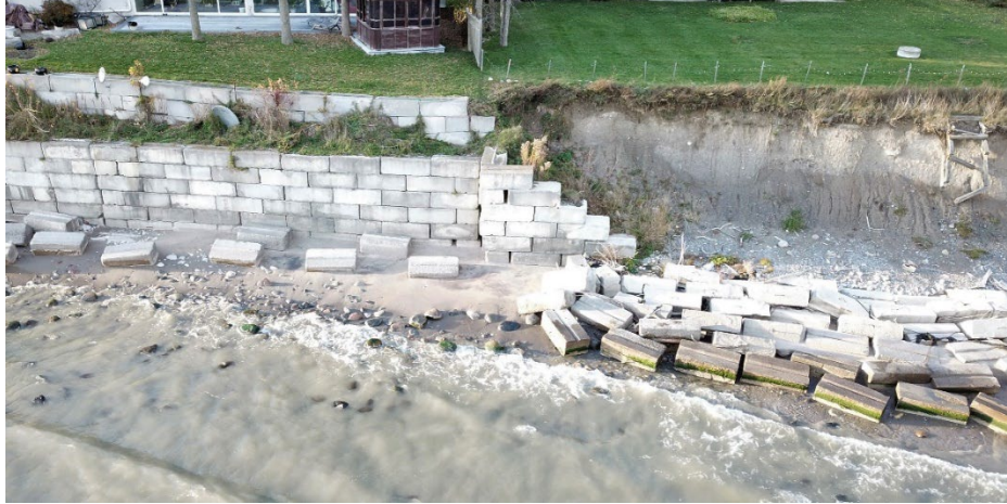
Figure 7.10 Failed vertical stacked concrete block seawall on Lake Ontario
