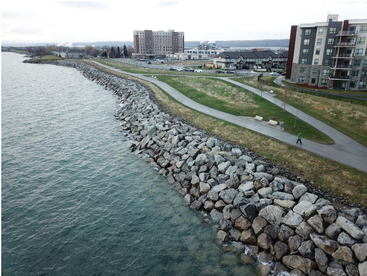
Figure 7.7 Conventional, multi-layer armour stone revetment on the HCA Lake Ontario shoreline
