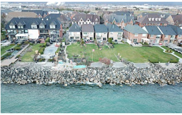
Continuous Shoreline Armouring at Edgewater Drive
