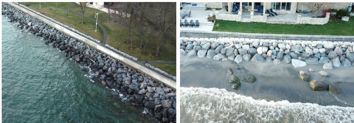
Figure 7.13 Examples of stone berms placed in front of vertical structures to reduce erosion at the toe, reduce wave reflection and overtopping, and provide added stability to the structure
