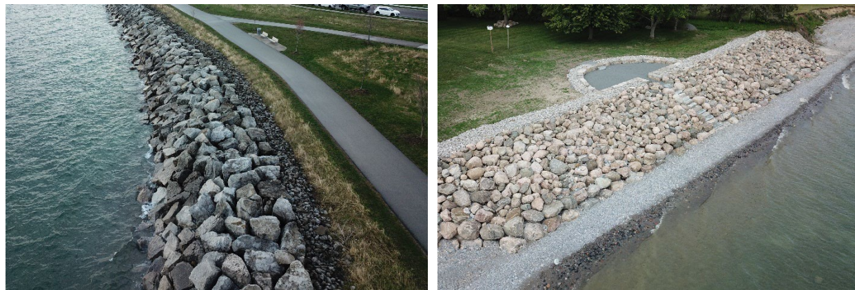
Figure 7.12 Examples of conventional, randomly placed, multi-layer armour stone revetments on the Great Lakes constructed with irregular armour stone (left) and field stone (right)
