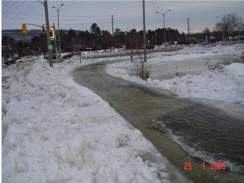
Figure 2-4: Temporary Overflow Channel at Dundas St. (Jan. 2005)
