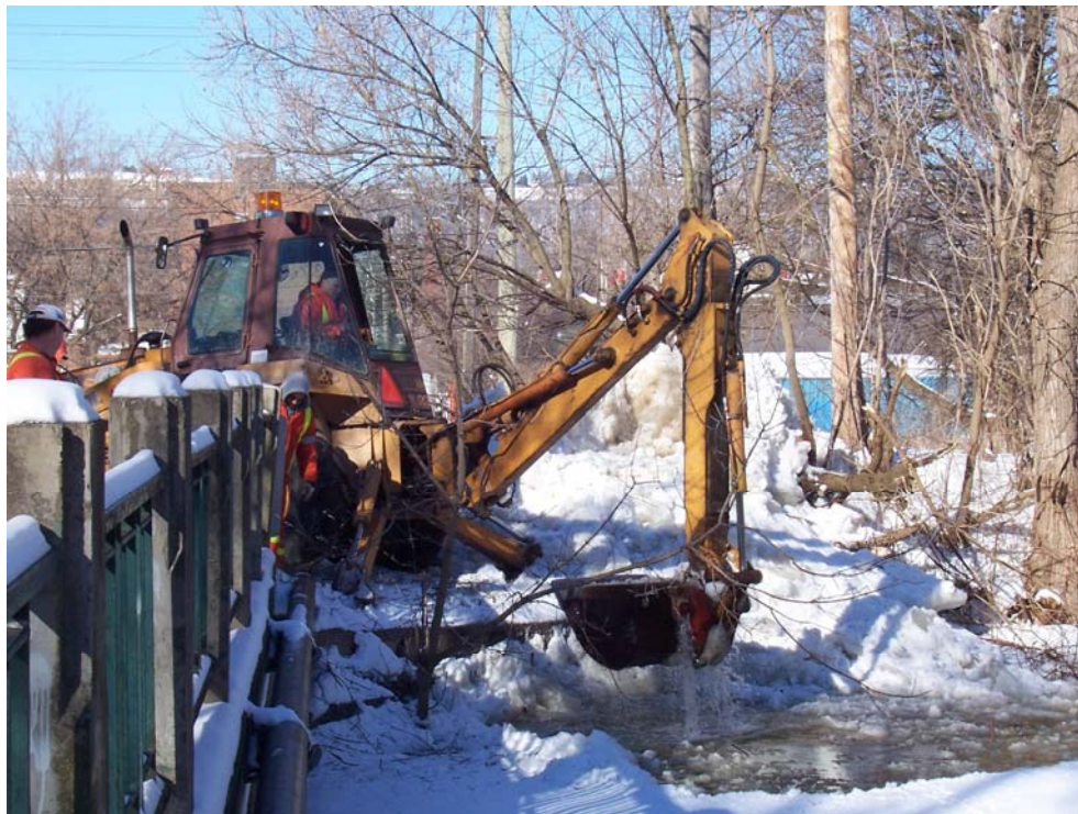
Figure 2-5: Mechanical Removal of Frazil Ice at Thorpe St. Bridge (Jan. 2005)
