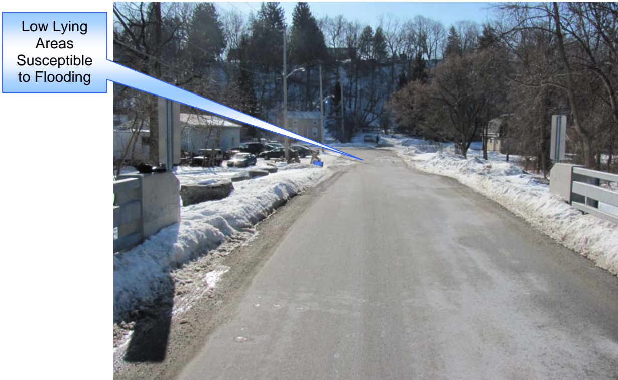
Photo 8: Looking South on Thorpe St., Feb. 15, 2011
