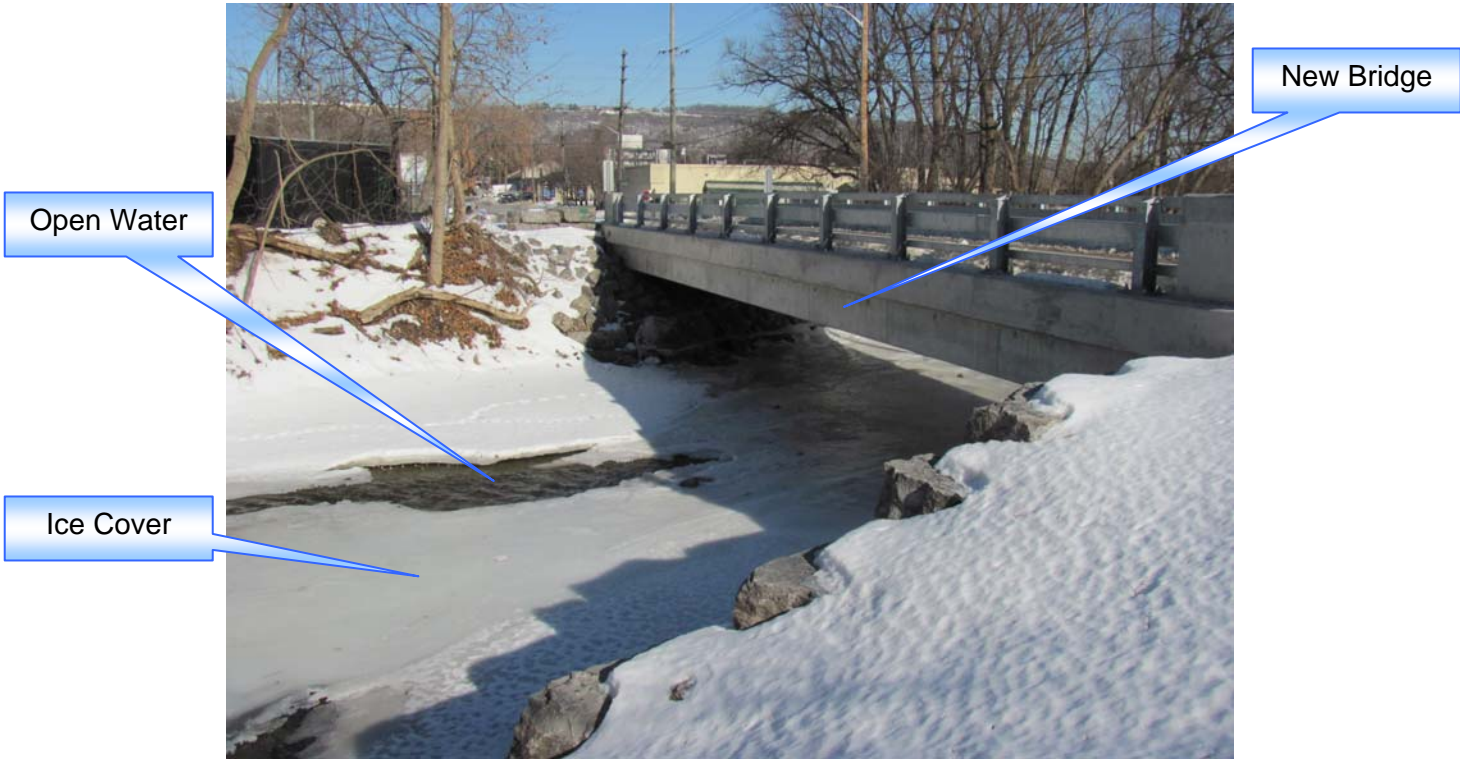
Photo 7: Upstream Side of the Thorpe St. Bridge, Feb. 15, 2011
