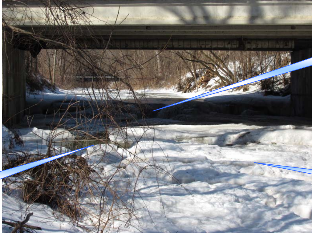
Photo 5: Step Weirs at Market St. Bridge, Feb. 15, 2011
