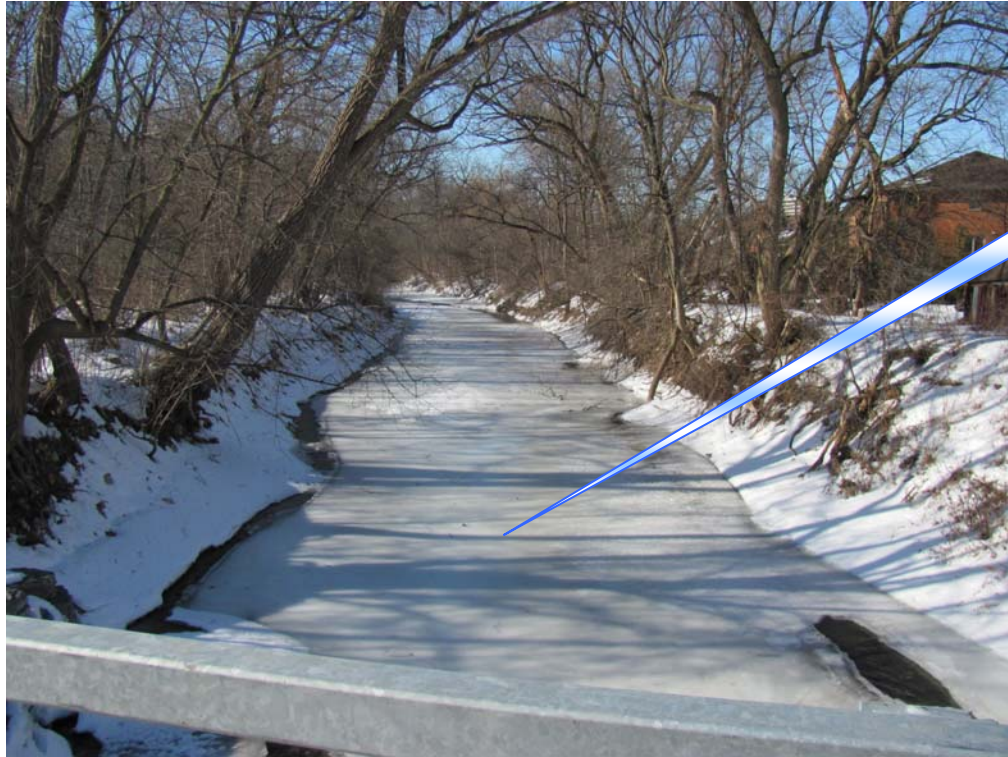
Photo 9: Upstream of Thorpe St. Bridge, Feb. 15, 2011
