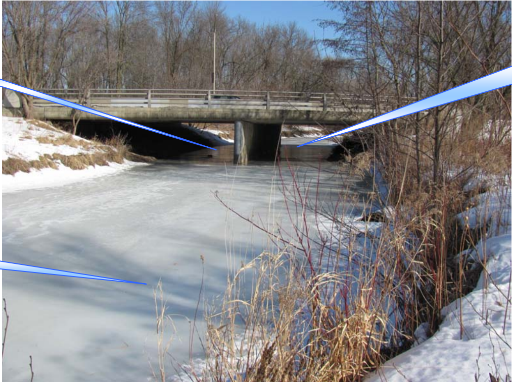
Photo 13: Upstream View of Cootes Dr. Bridge, Feb. 15, 2011
