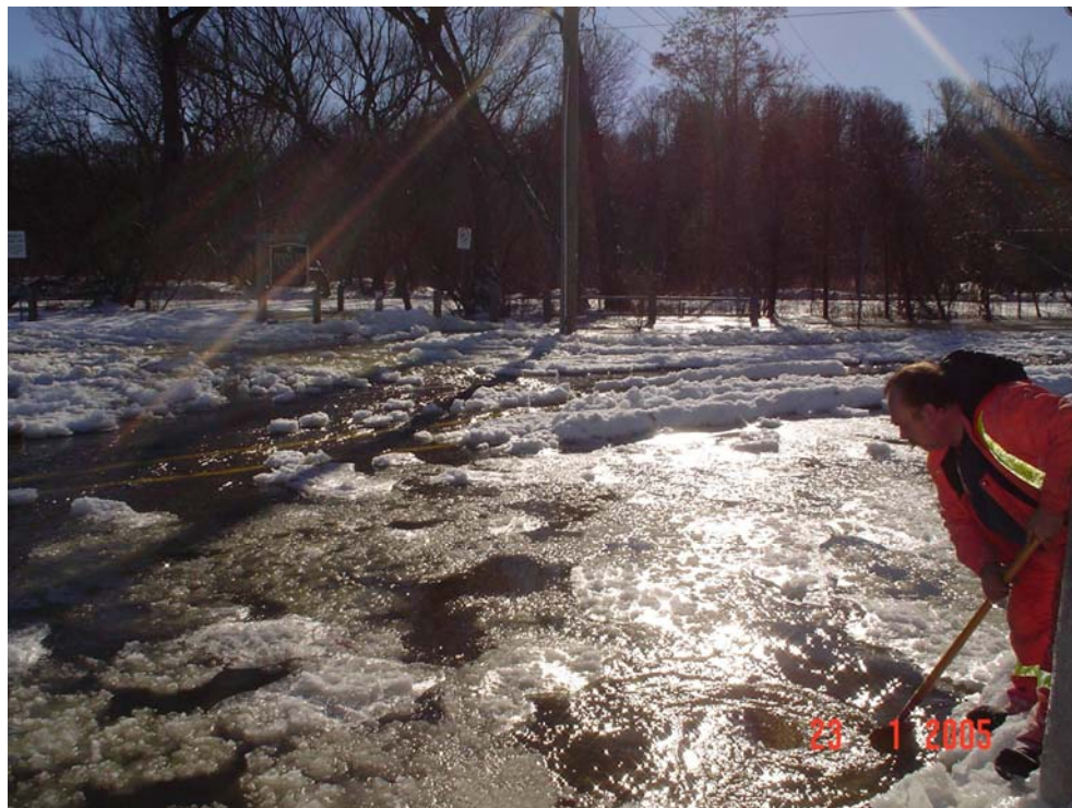
Figure 2-3: Clearing Catchbasins on Dundas St. (Jan. 2005)
