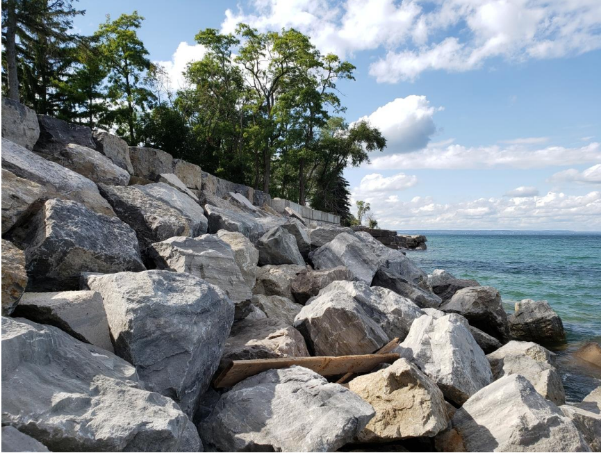
Photo 3 – Shoreline of Subject Property (looking west)
