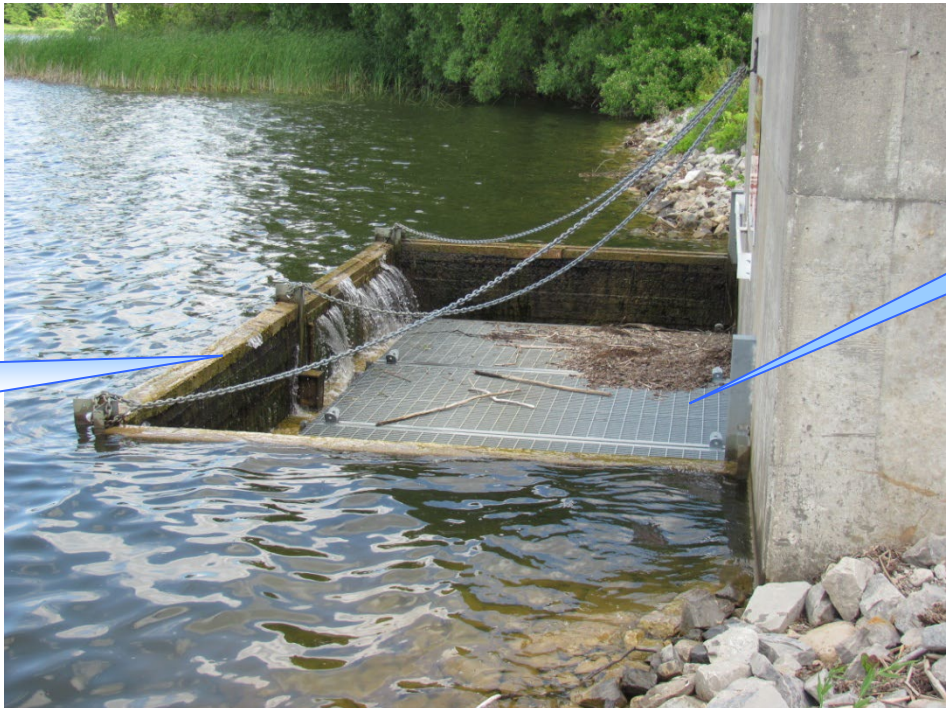
Photo 8: Drop inlet structure (July 2011)
