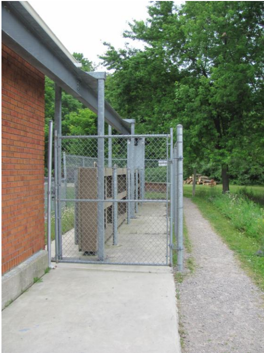
Photo 17: Steel panels storage area (July 2011)
