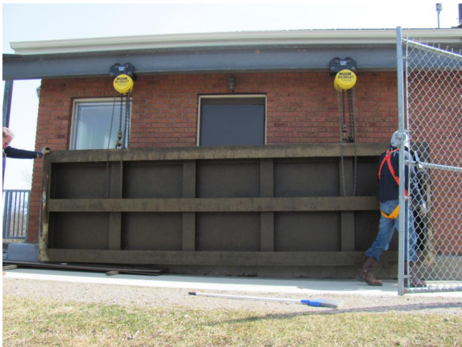
Photo 16: Transporting the steel panels (April 2011)
