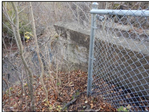
Photo 43 – End of Exterior Fencing
