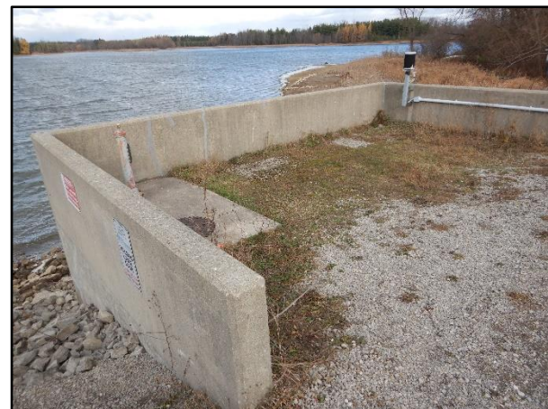
Photo 18 – Inlet Structure Barricade
