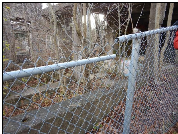
Photo 45 – Exterior Fencing Deficiency
