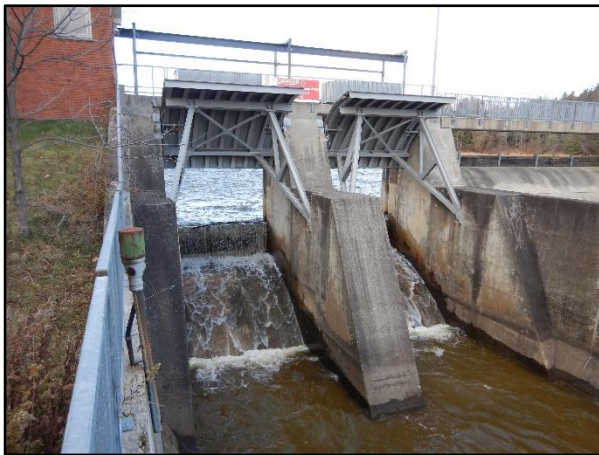
Photo 5 – Main Spillway Gates
