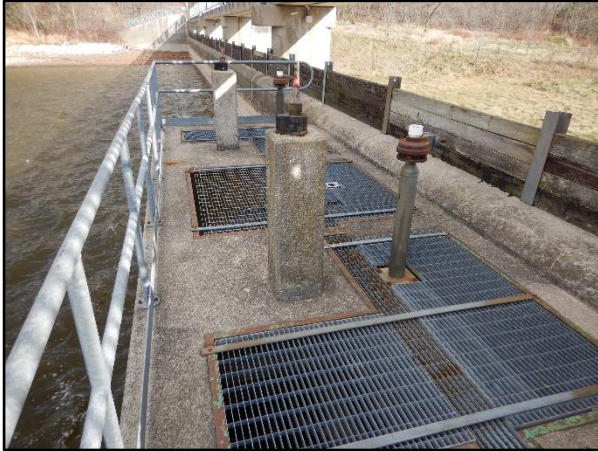
Photo 9 – Drop Inlet Structure Deck
