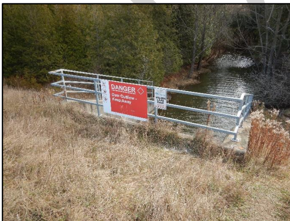
Photo 17 – Outlet Structure Railing
