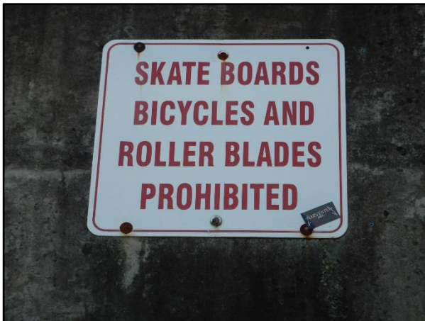
Photo 29 – Public Safety Sign on Right End of Overflow Weir
