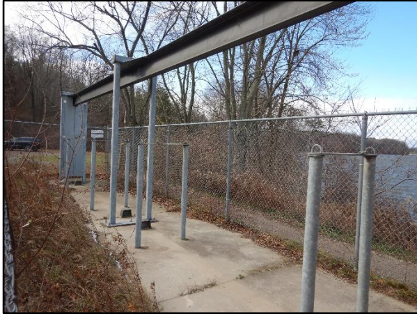
Photo 27 – Storage Area for Winter Gate Panels
