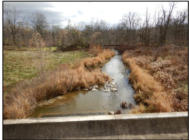
Photo 12 – Low Flow Channel
