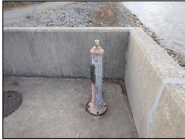
Photo 6 – Low Flow Valve Stem
