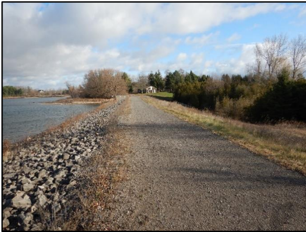
Photo 1 – Access Road Across Dam
