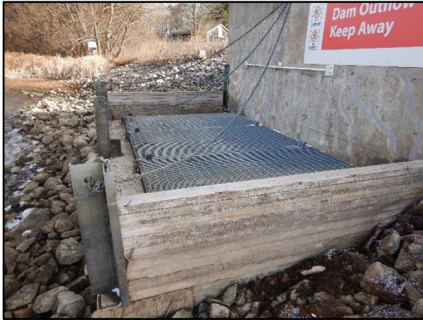
Photo 5 – Concrete Inlet Structure
