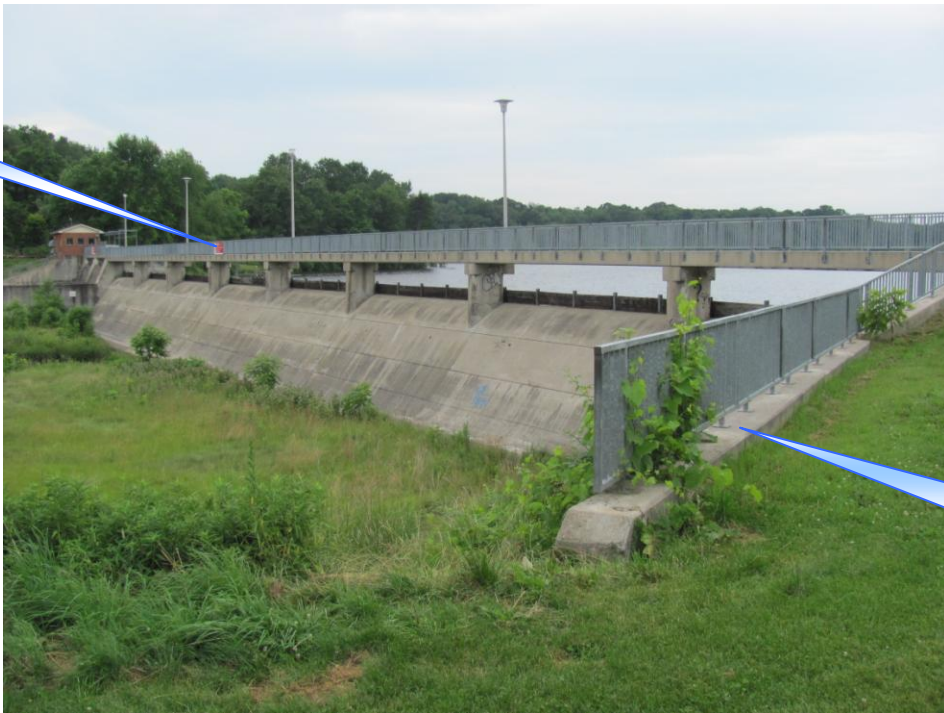
Photo 8: View of downstream face of ogee weir (July 2011)
