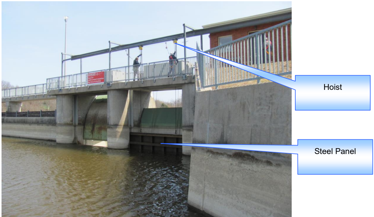
Photo 16: Transporting the steel panels (April 2011)
