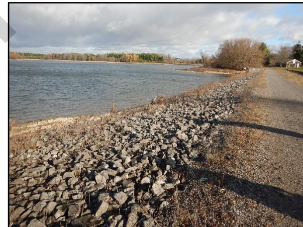
Photo 4 – Upstream Earth Embankment
