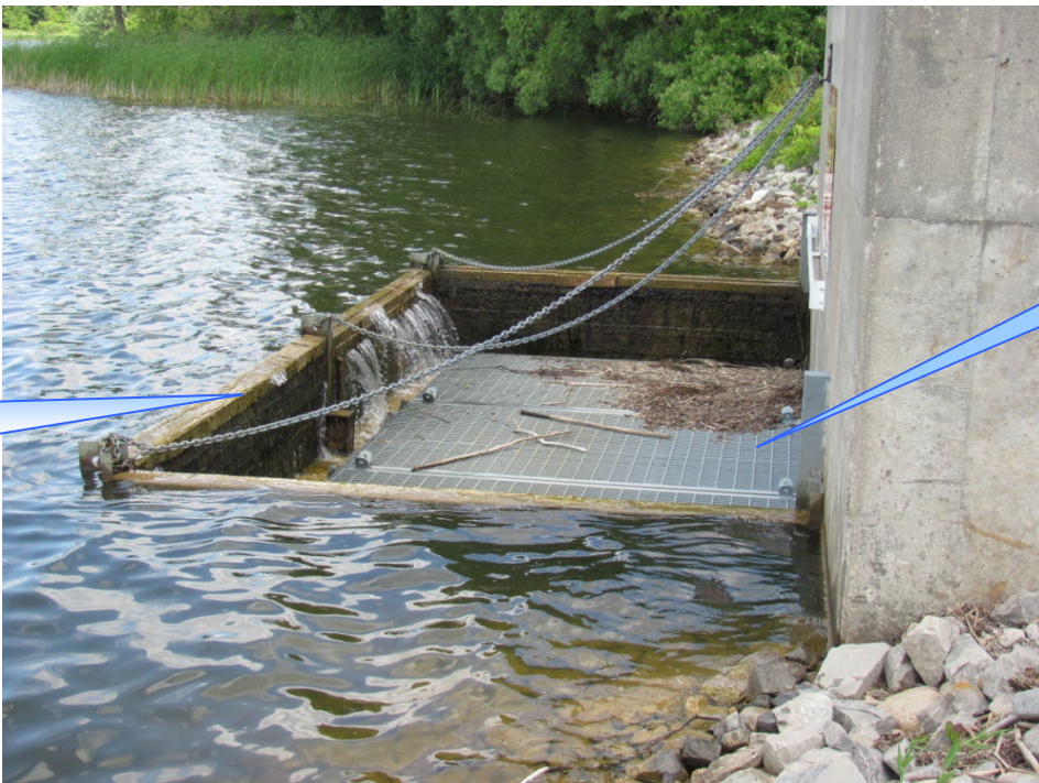
Photo 8: Drop inlet structure (July 2011)
