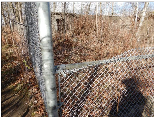
Photo 44 – Exterior Fencing Deficiency (Possible Evidence of Fence Climbing)
