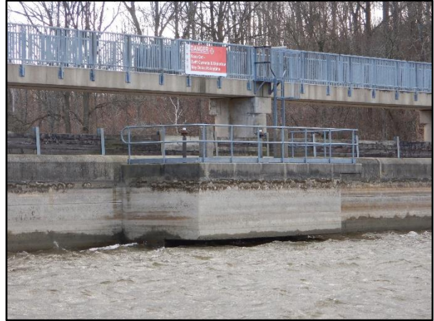
Photo 10 – Drop Inlet Structure
