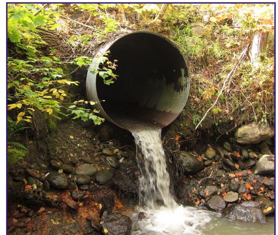
Perched Culverts and On-line Ponds Limit the Movement of Fish
