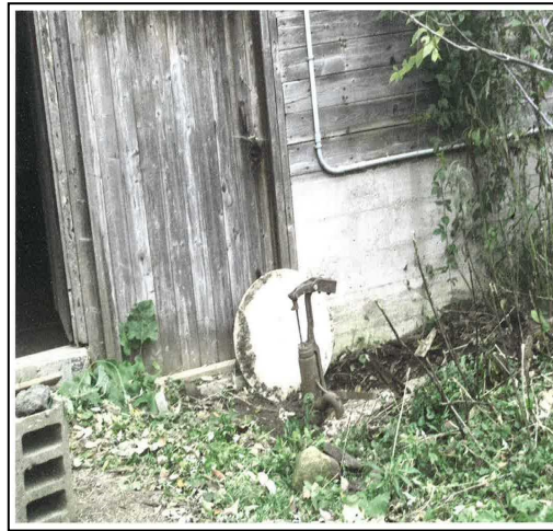
Before Well Decommissioned
