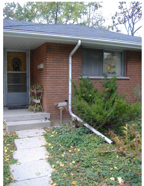
Disconnected downspout allows precipitation to infiltrate the soil.
