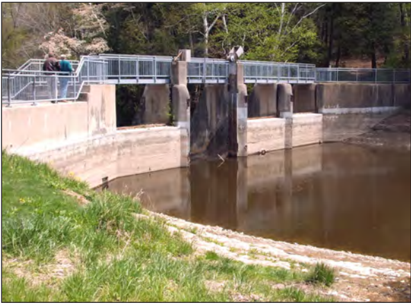
Upstream face of dam.
