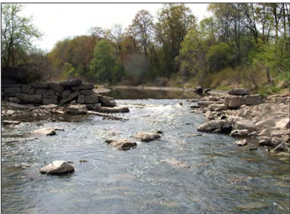
View of remnant Mill Dam at mid-point in reservoir.
