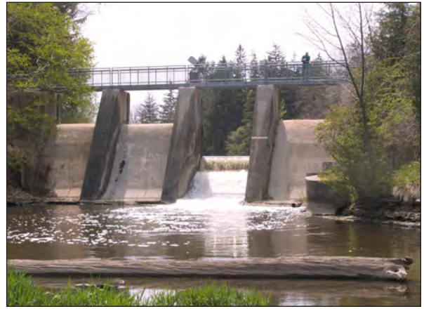
Downstream face of dam.
