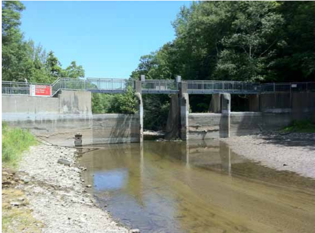
Figure 2-1 A View of the Upstream Face of Crooks' Hollow Dam Showing Concrete Wear and Cracking
