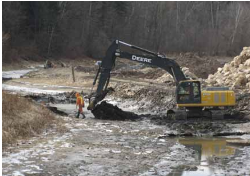
Figure 5-3 Sediment Being Excavated from the Creek Bed During Construction Activities
