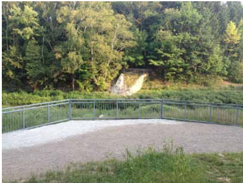
Figure 5-13 Remaining Dam Abutment and Lookout Areas Created to Preserve Cultural Heritage (View from Northern Bank, Opposite Crooks' Hollow Road)
