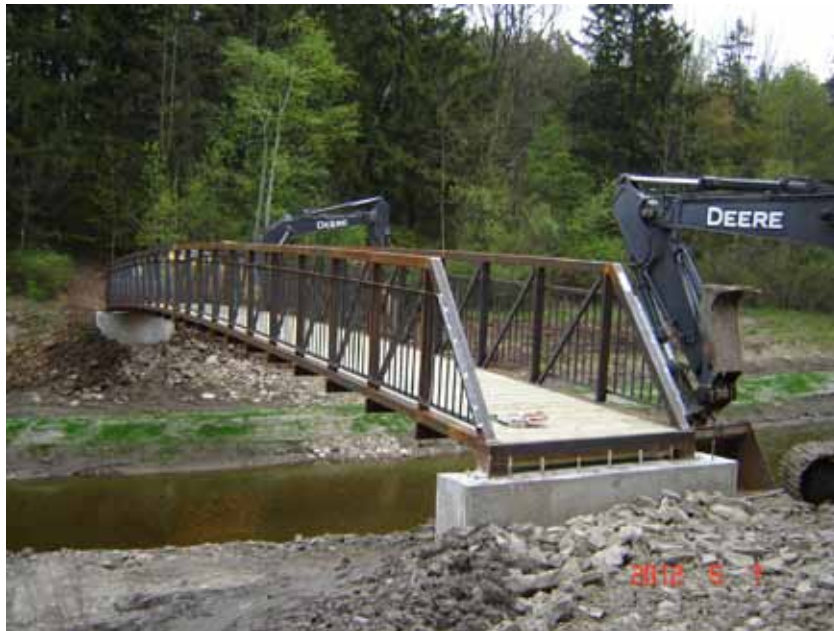
Figure 5-10 Construction Workforce Finalizing Pedestrian Bridge Installation
