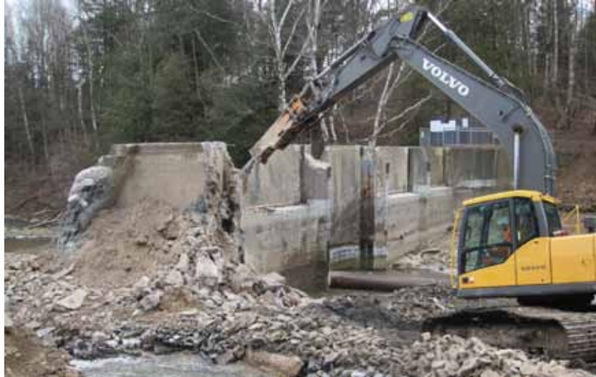
Figure 5-9 Excavator Breaking Up Dam Structure with Hoe-Ram
