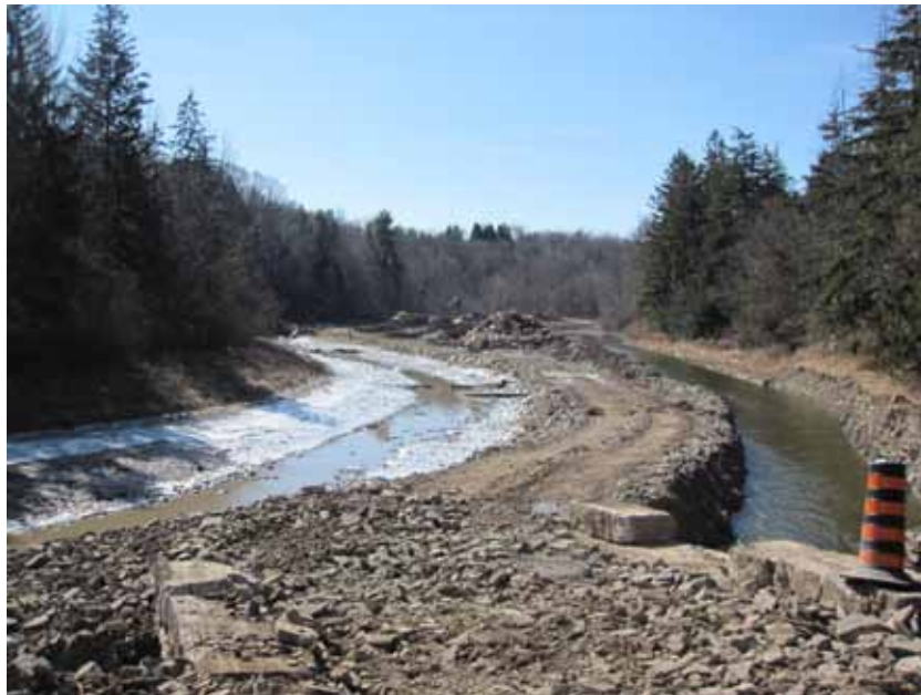
Figure 5-1 Diversion Channel (Right Side) Created to Facilitate Construction and Dam Decommissioning Activities
