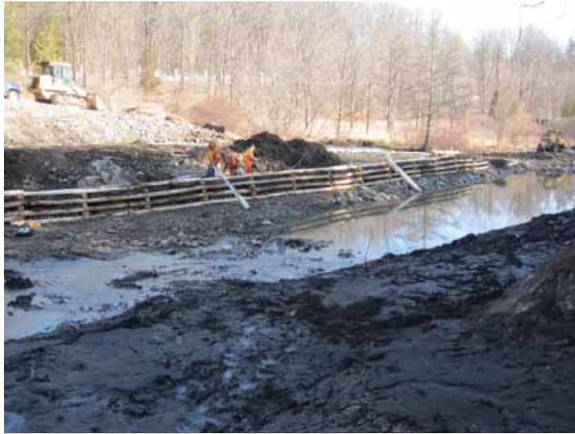
Figure 5-8 Construction of Crib Wall Downstream of Former Dam Site
