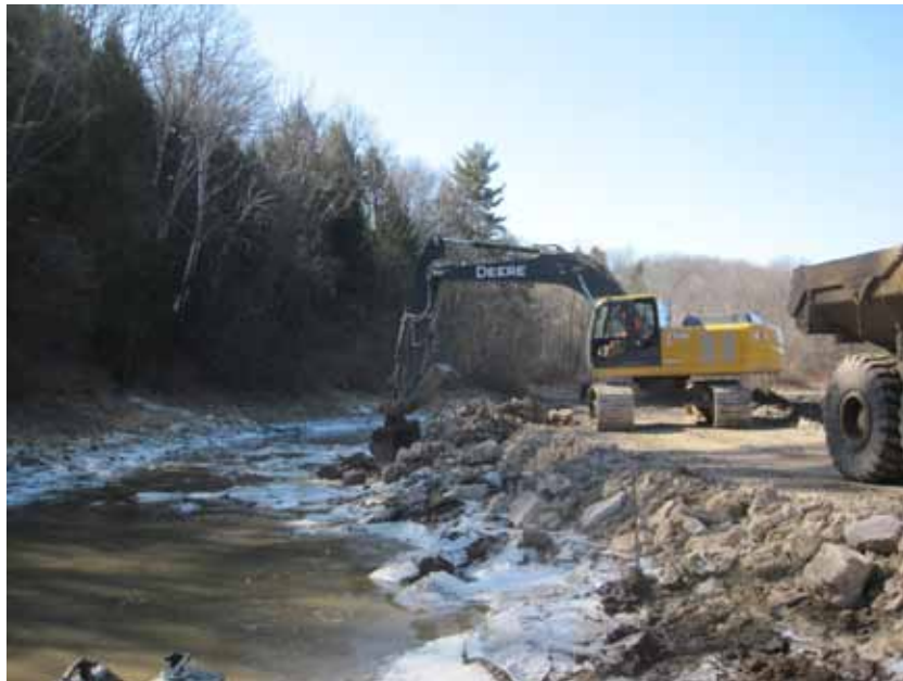
Figure 5-7 Construction of a Riffle Area Upstream of Former Dam Site
