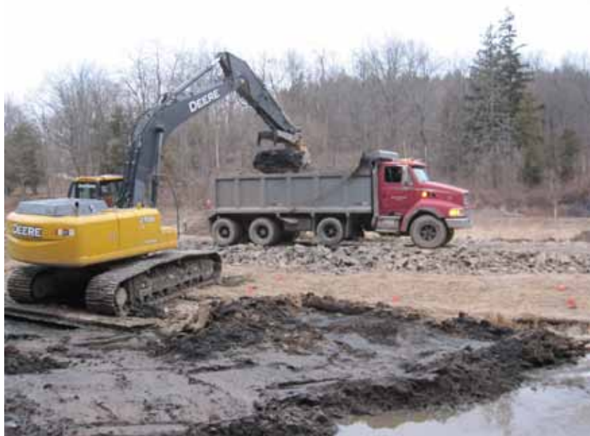
Figure 5-5 Mercury-Impacted Sediment Being Excavated from Creek Bed and Taken Offsite for Safe Disposal
