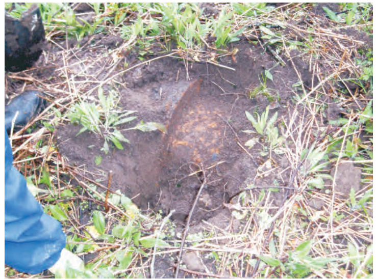
Plate 10 Close-up of Test Pit with Exposed Cast Iron Conduit
