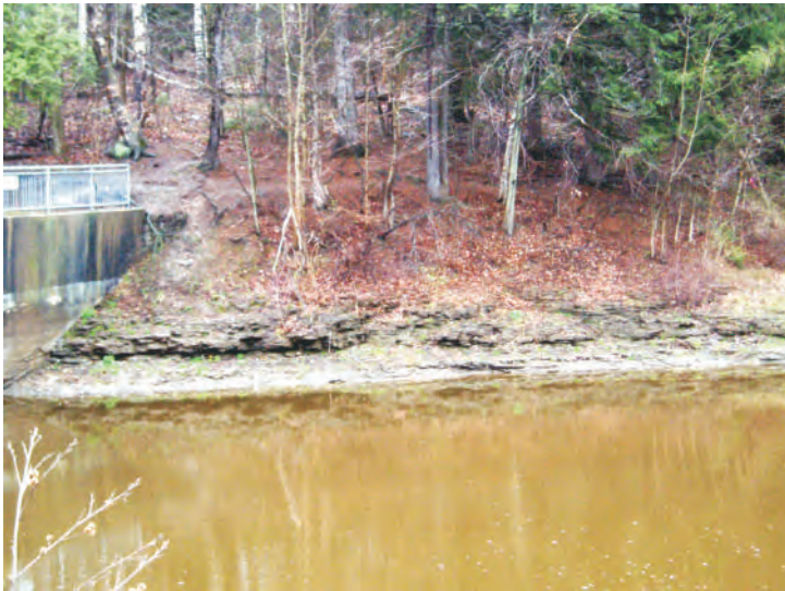
Plate 7 Crooks' Hollow Dam, View to Slope and Bedrock on the South Bank of the Creek
