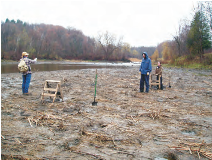
Plate 3 Test Pitting the Mud Flats, View Upstream
