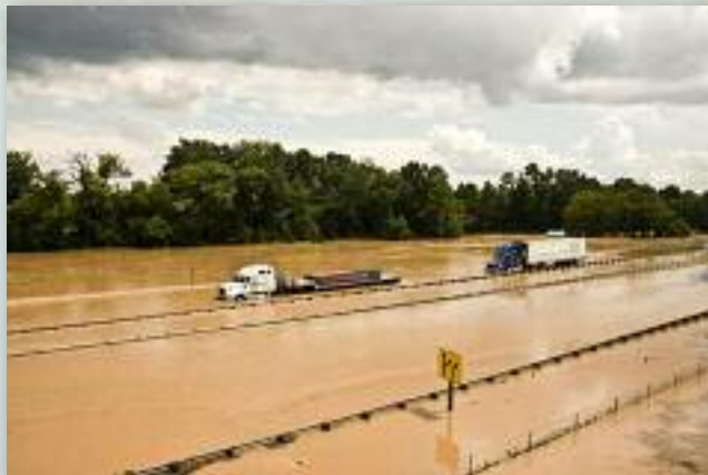
Flooding on Red Hill Valley Parkway (July 26, 2009) Photo Courtesy of Hamilton Spectator
