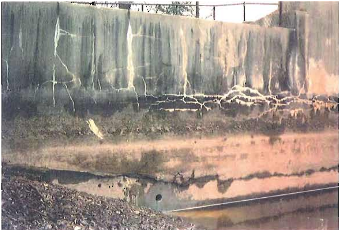
Photograph No. 2 - Upstream face of North Abutment.
