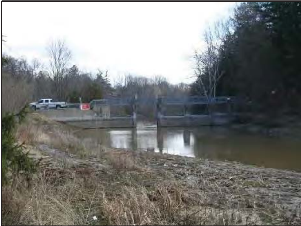
Plate 19: Drained reservoir above dam
