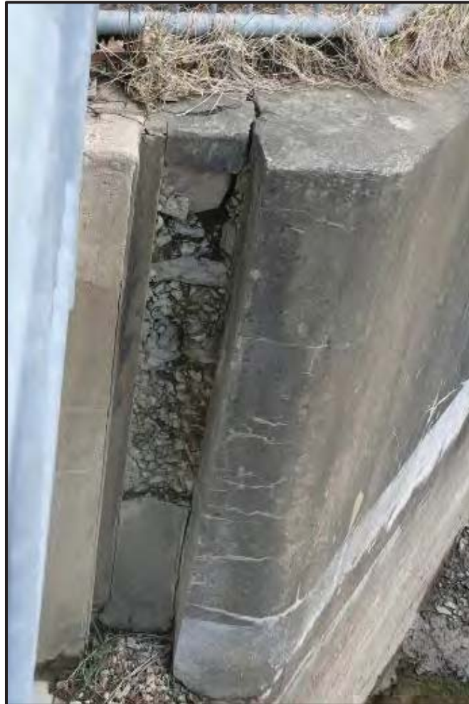
Plate 11: Large gravel evident in concrete visible in stop log slot of Spillway 4
