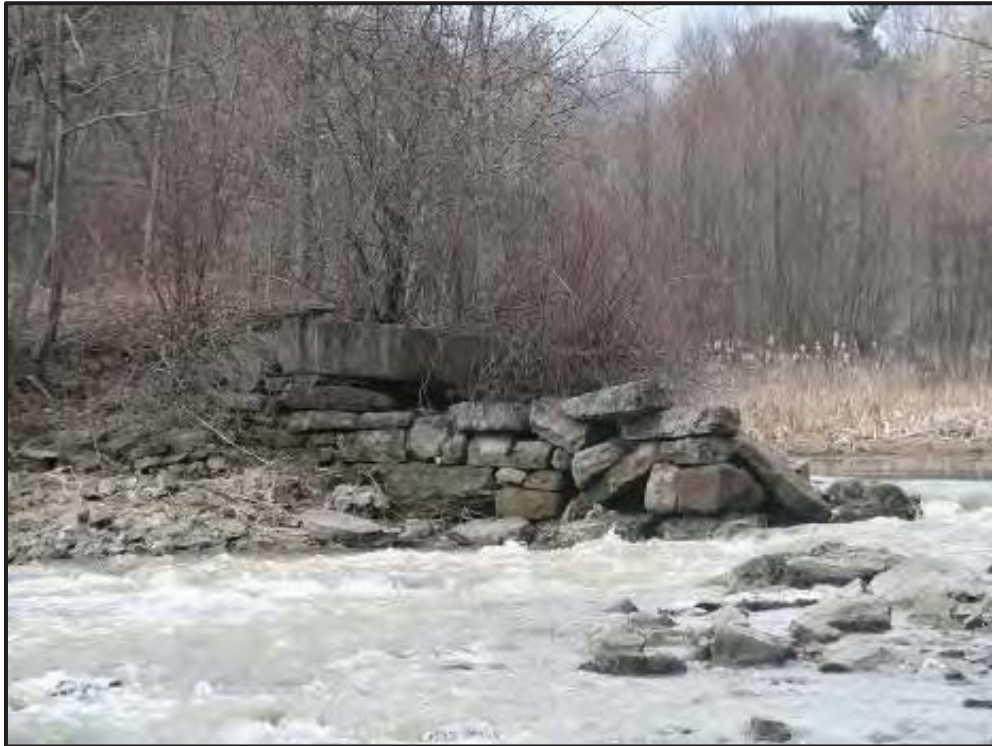
Plate 15: Detail of stone blocks in the weir as it is attached to the dyke on the south bank.
