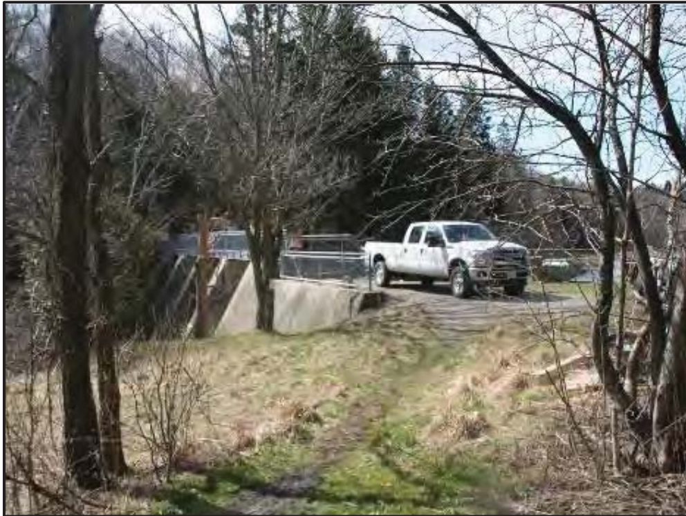
Plate 9: Concrete and earth abutment on west side of dam
