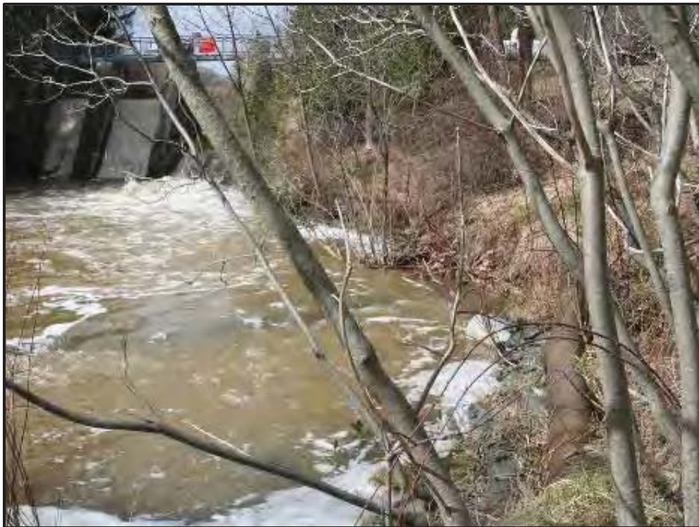
Plate 13: Iron conduit along bank of Spencer Creek with dam in rear
