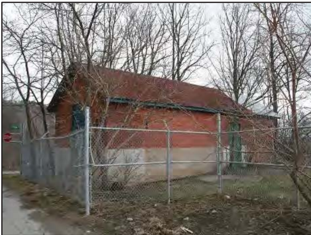
Plate 2: Pump house at the Dundas reservoir in 2011
