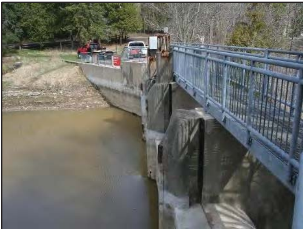
Plate 10: Dam crest, and stop log slot, earth berm and bridge looking to west bank
