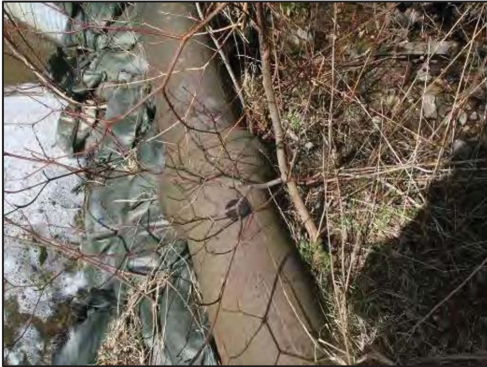
Plate 12: The cast iron water conduit was laid on the ground adjacent to the creek rather than buried
