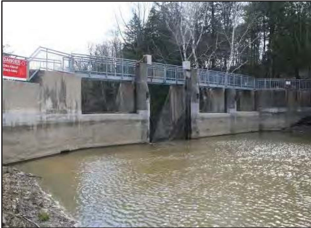
Plate 7: Upstream View of Dam looking to east abutment. The low #2 spillway is evident as are the buttresses that could increase the depth of the reservoir if needed. The metal footbridge provides a public crossing of the stream.
