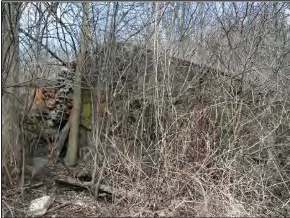
Plate 18: South end of Cockburn Mill dam concrete weir. The earth dam across Spencer Creek would have extended to the left of this structure. The rock filled crib construction is visible in the end of the weir.
