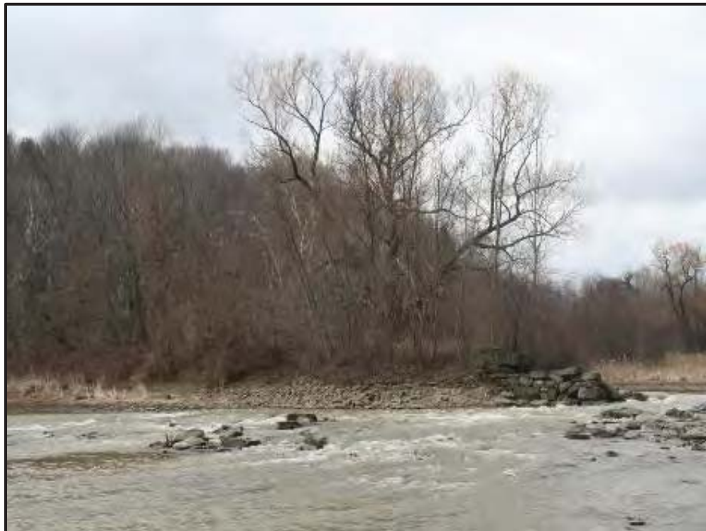
Plate 14: Looking upstream to the dam at Morden Mill
