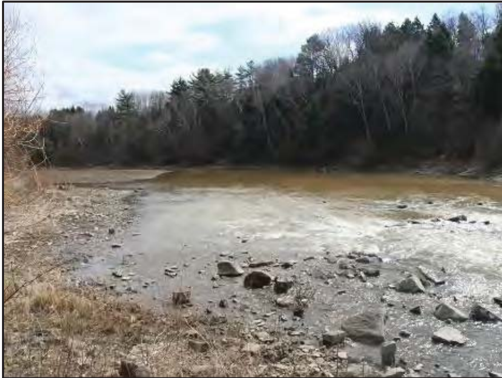
Plate 21: Looking downstream over reservoir at Morden Mill Dam
