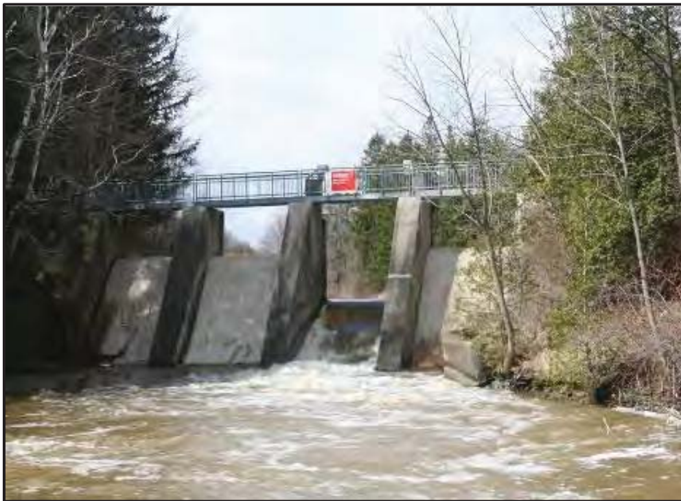
Plate 8: Looking upstream to Dam showing lower level of Spillway 2 crest
