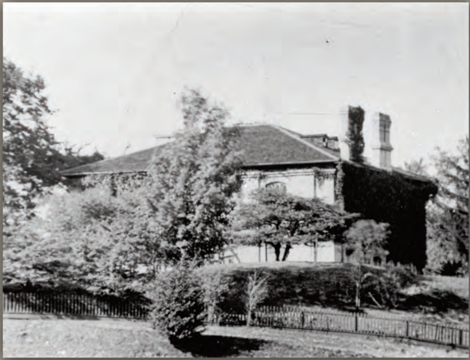
In 1855, The Hermitage was purchased by George Leith. When The Hermitage mansion was completed, it was used basically as a summer home. Most winters were spent in Hamilton or even Scotland.
